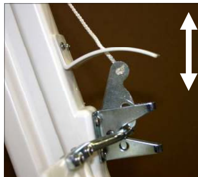
Step 6: Pull finger ring numerous times to check for proper gate latch operation. It is extremely important that gate latch closes properly & freely over striker bar. Secure with lock
